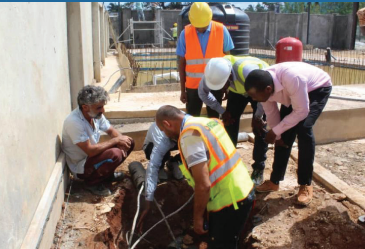
Fiber Expert team inspect existing Route at New Amani Stadium.
